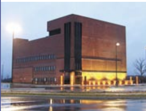
MMCIC has invested $3 million to prepare the building at 460 Capstone Circle, plus adjacent roadways and parking lots, for the consolidated dispatch center. About 100 employees will work there.
