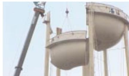
**CH2M Hill dismantled and shipped this water tower to another location to be reassembled and reused.**
